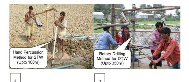
Figure 4.3: Irrigation wells are relatively inexpensive, easy to install using local methods, as well as easy to maintain that leads to uncontrolled installation of wells
